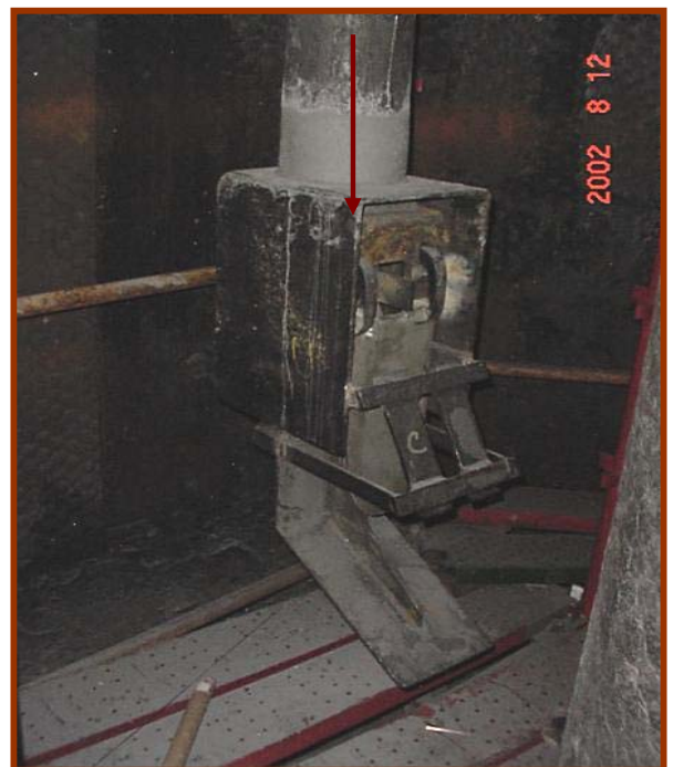
Fig. 11 Completed repair area
