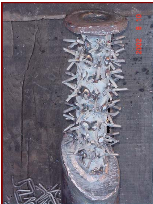
Fig. 13 – Nozzle with Vee Anchors
