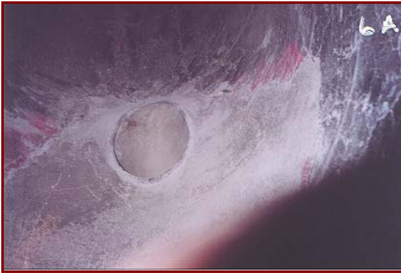
Fig. 06 Post Dry-Out Photograph
