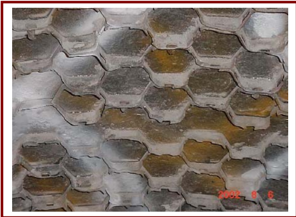
Fig. 01 Hexmesh on Cyclone Roof after removal of refractory
