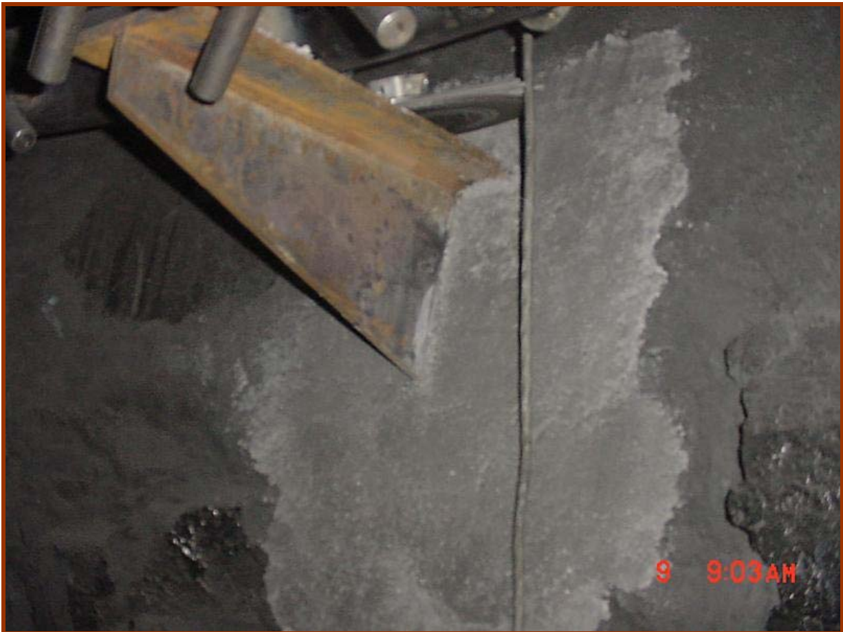
Fig. 14 – ACTCHEM (grey material) packed onto single point anchors
